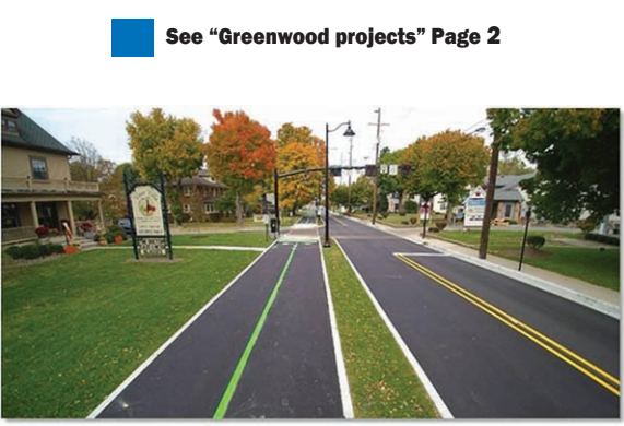
Portion of completed Madison Avenue streetscape shows walking trail on west side and sidewalk on east side, similar to the third phase with construction to begin soon to Fry Road.
