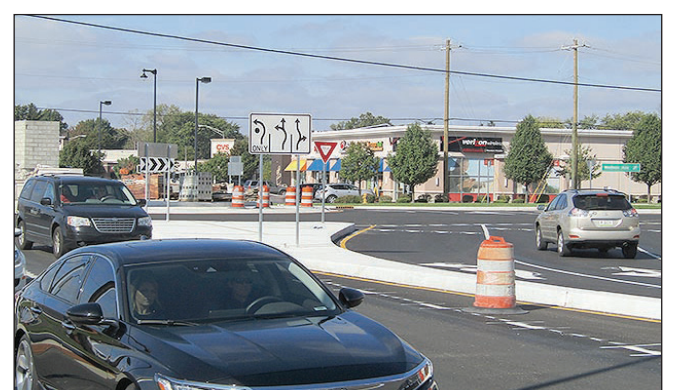
Westbound motorists on Smith Valley Road have this view of the new roundabout to be used to reach Madison Avenue or U.S. 31 or to continue west across U.S. 31.
