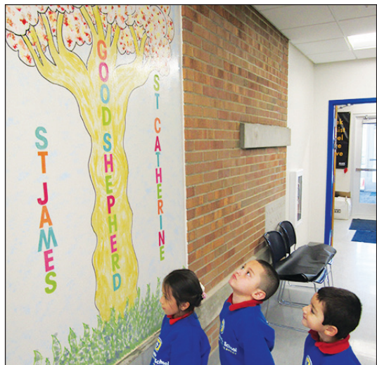
Central Catholic pre-k students, from left, Emily Mendova, Benito Delgado and Gael Romero-Vidal admire one of two paintings on the old exterior north wall that is an interior wall after completion of two new classrooms and a secure main entrance.
